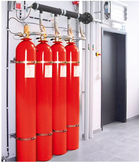
Sinorix 227 provides fast, efficient extinguishing without residues.
